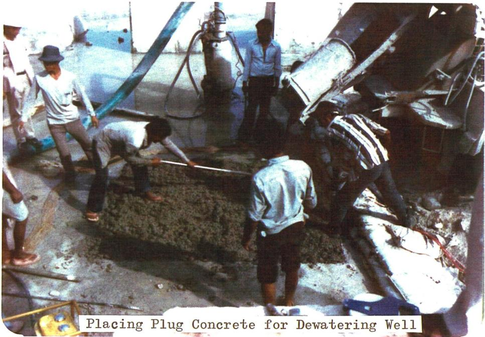
Placing Plug Concrete for Dewatering Well
