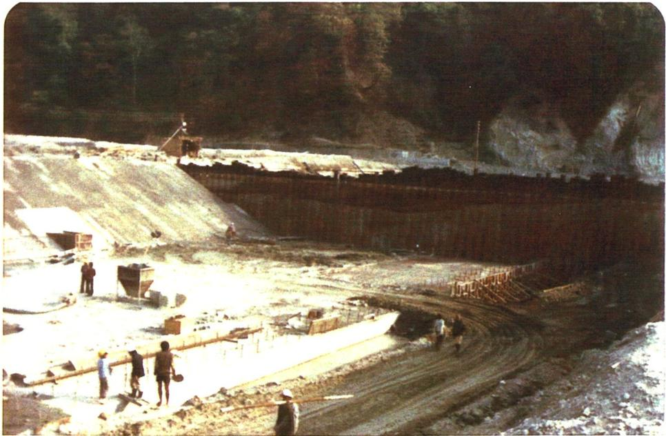
Completion of Placing Concrete for Right-half of Stilling Basin
