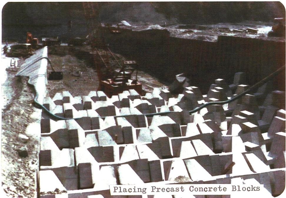
Placing Precast Concrete Blocks
