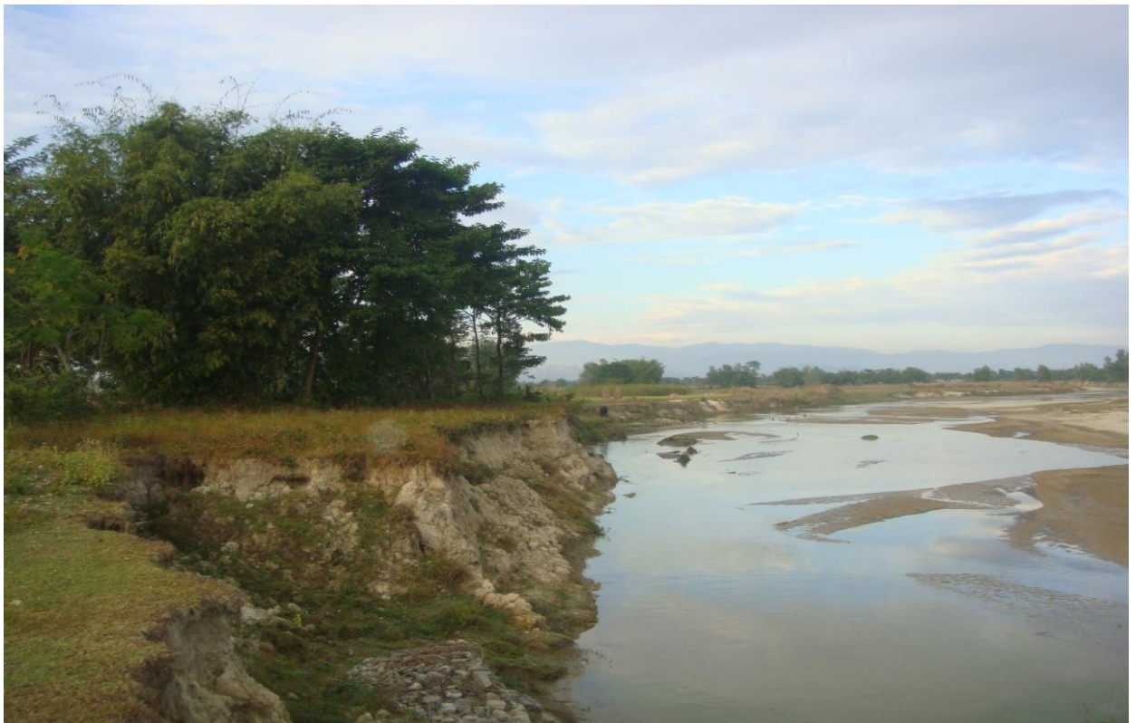
Kamal river flowing parallel near main canal and damaging the bank of canal at ch. 11+000.
