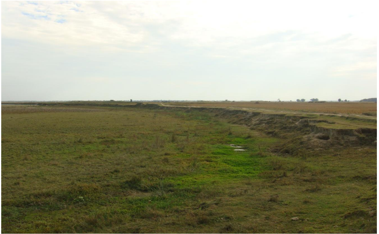
Canal washed out about 200 meter length by flood of S12 at chainage 4+900.
