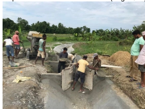
Construction of Water Measuring Device (Parshall Flume) (Jun. 2022)
