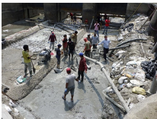
Repair of Headworks Concrete Casting at Upstream of Scouring Gate
