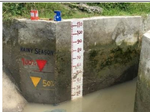
Marking of Discharge Water Level Discharge Water Level in Rainy Season at SC-0
