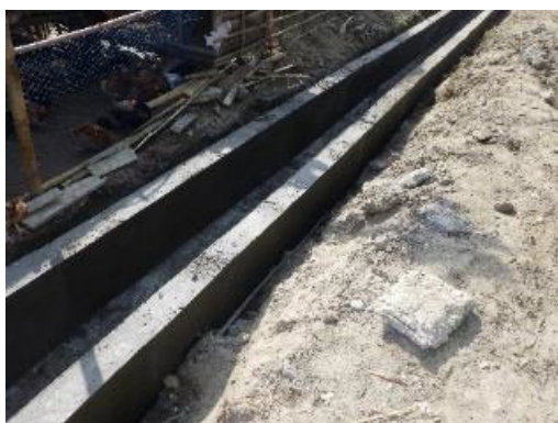
Constructed Concrete Flume Canal in TC
