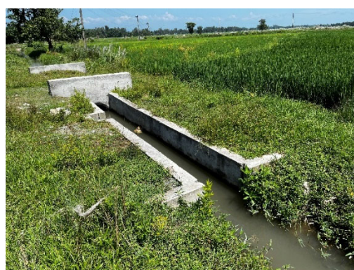
Constructed Field Outlet with Road Crossing
