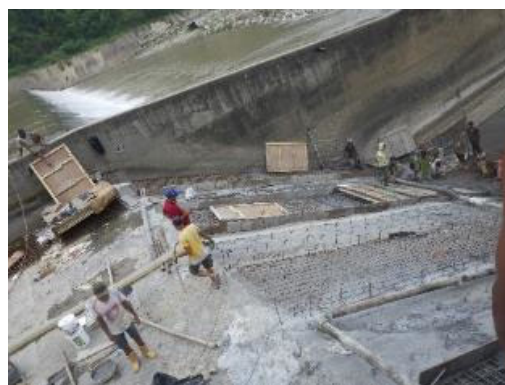
Repair of Headworks Concrete Casting at Shoot
