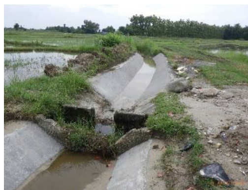
Constructed Concrete Lining of TC
